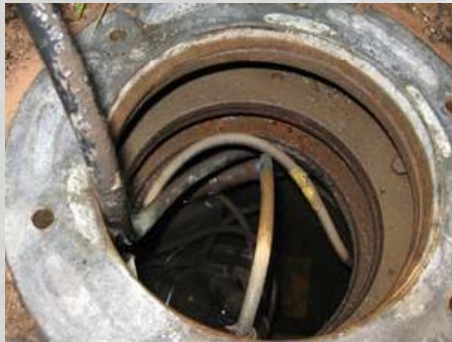
Water Accumulation in Base Can
