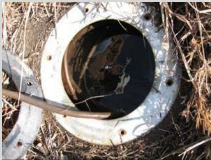
Water Accumulation in Base Can
