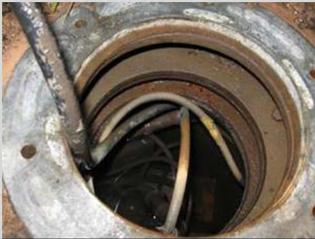
Water Accumulation in Base Can
